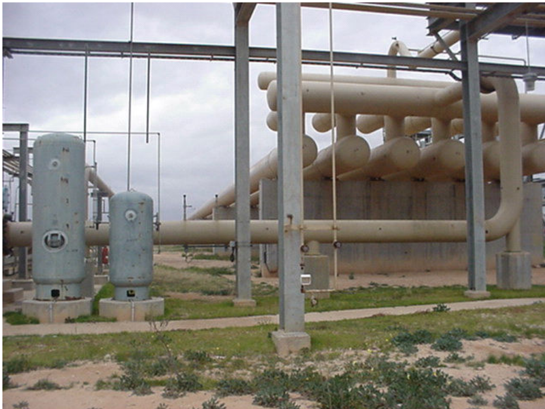
Figure 10: Multi-pipe slugcatcher at the BG Hannibal Terminal showing the inlet pipe and header, and the short separation fingers above the much longer liquid fingers.
